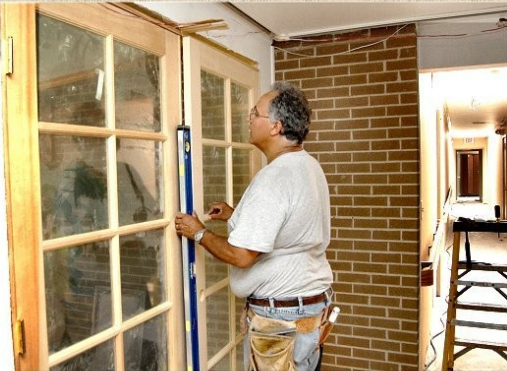
LEVELLING WITH THE FRENCH DOORS
